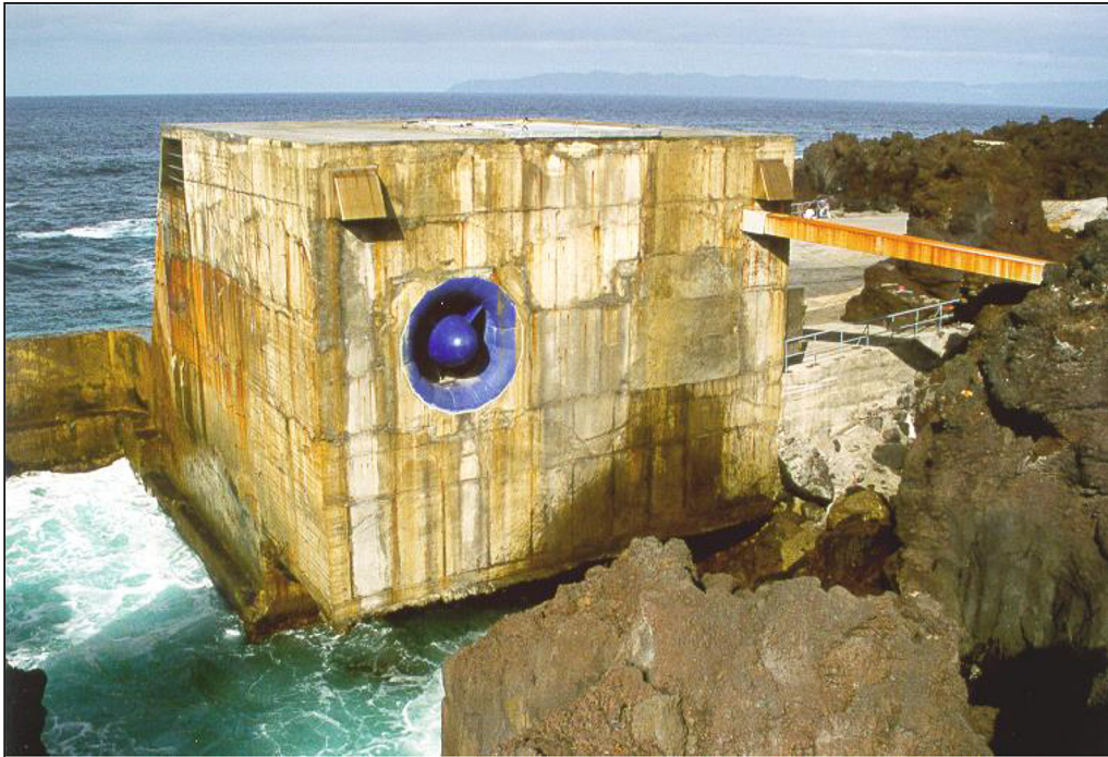
Fig. 10. Back view of the 400 kW OWC plant on the island of Pico, Azores, Portugal, 1999.
