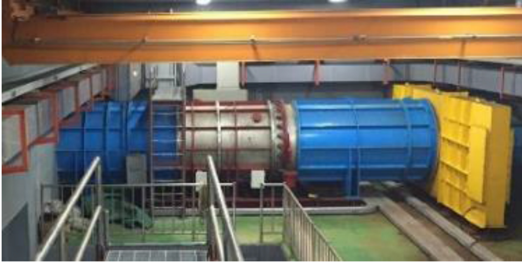
Fig. 42. One of the two 250 kW impulse turbines of the bottom-standing OWC plant at Jeju Island, South Korea.
