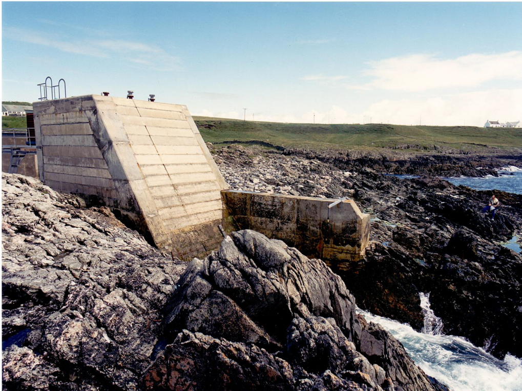
Fig. 6. Shoreline OWC on the island of Islay, Scotland, rated 75 kW, commissioned in 1991 (courtesy of M. Folley).
