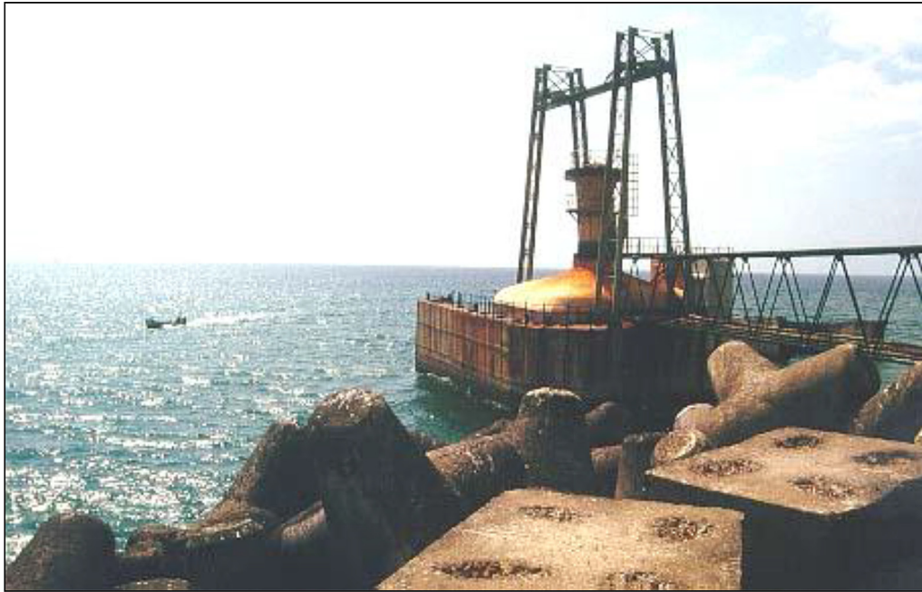
Fig. 8. Bottom-standing OWC installed in 1990 at Trivandrum, southern India. Rated power 125 kW.
