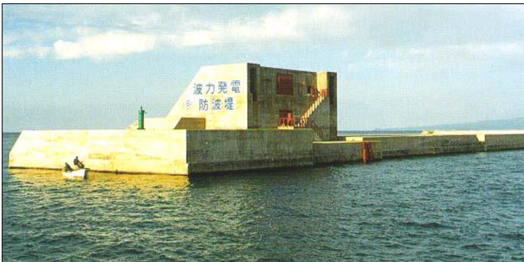
Fig. 7. OWC plant integrated into a breakwater at Sakata harbour, Japan, 1990. Rated power 60 kW.
