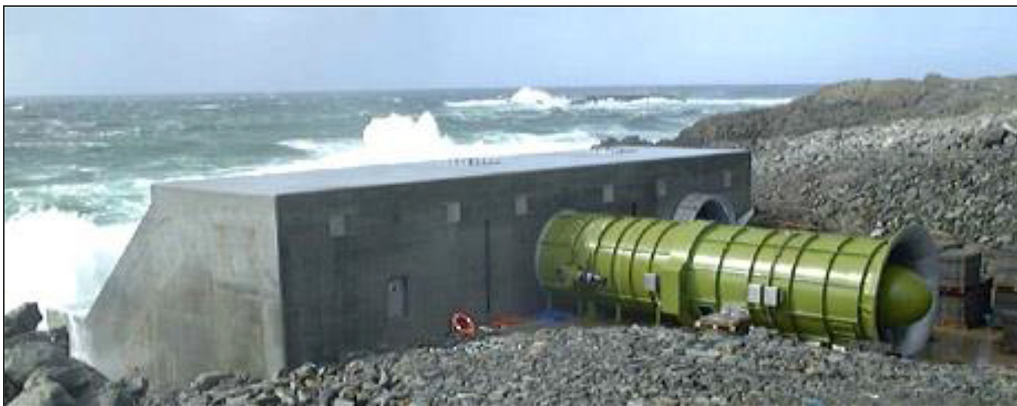
Fig. 11. LIMPET OWC plant, rated 500 kW, installed in 2000 on the island of Islay, Scotland, UK.
