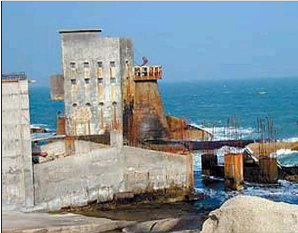
Fig. 12. 100 kW shoreline OWC built in 2001 in Guangdong Province, China [27].
