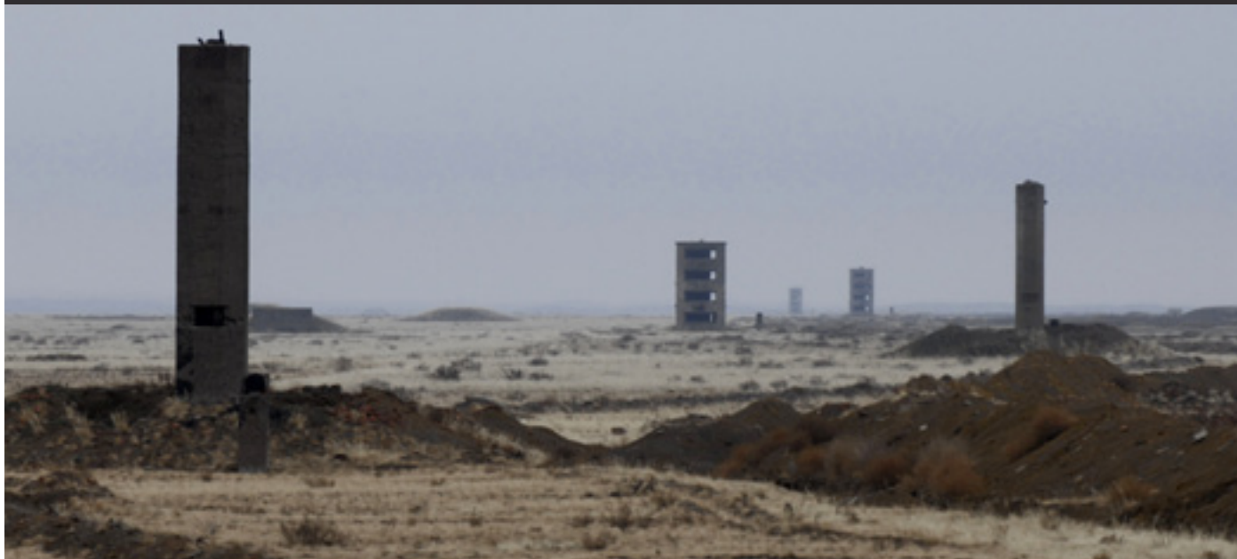
Bunkers that housed measuring devices and instruments near Ground Zero at the Semipalatinsk Test Site in Kazakhstan. Even today, more than 20 years after the last test was conducted, vast areas remain uninhabitable and unsuitable for productive use. Photo: John Van (Scanpix)
