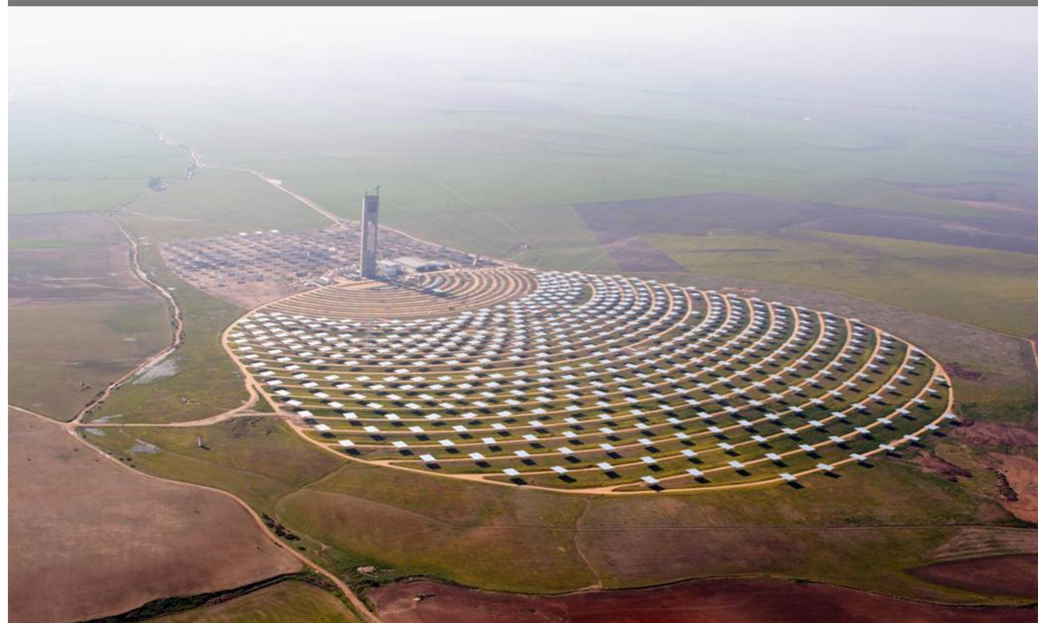
Abengoa started the developments in this field during **1984** taking part in the construction of **Plataforma Solar de Almería**. For that Abengoa built various compounds, like **heliostats and facets**, and assembled several equipments in the Cesa tower.
