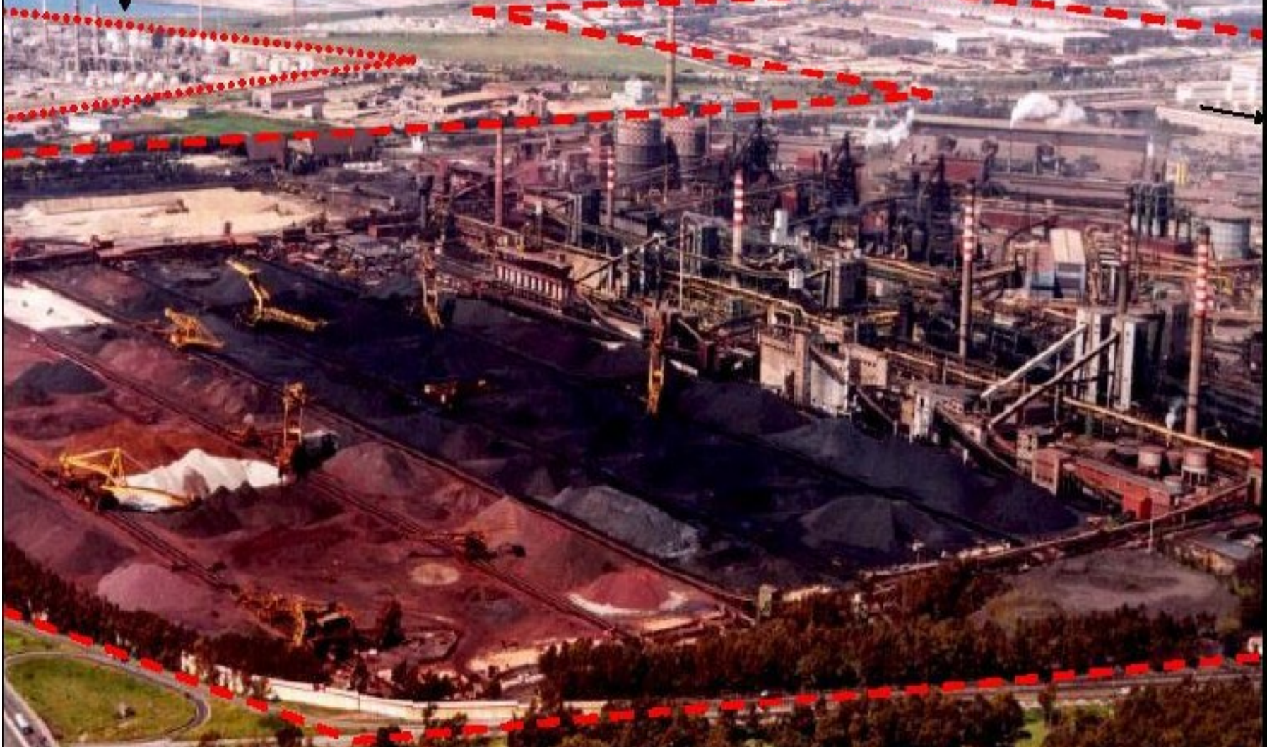
INTEGRATED IRON AND STEEL PLANT TARANTO
