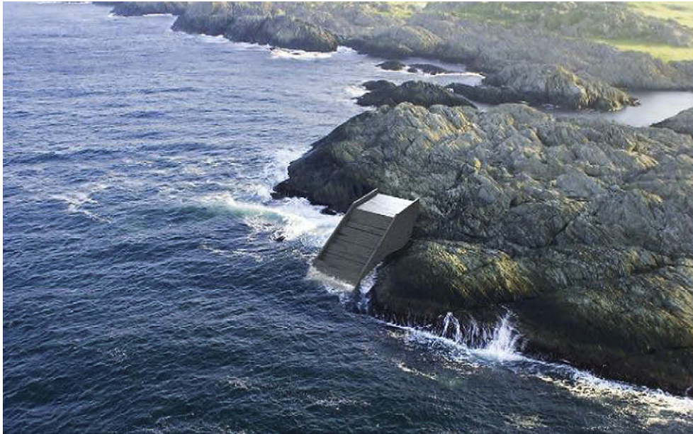
Fig. 1. The SSG pilot plant in the island of Kvitsøy, Norway.
