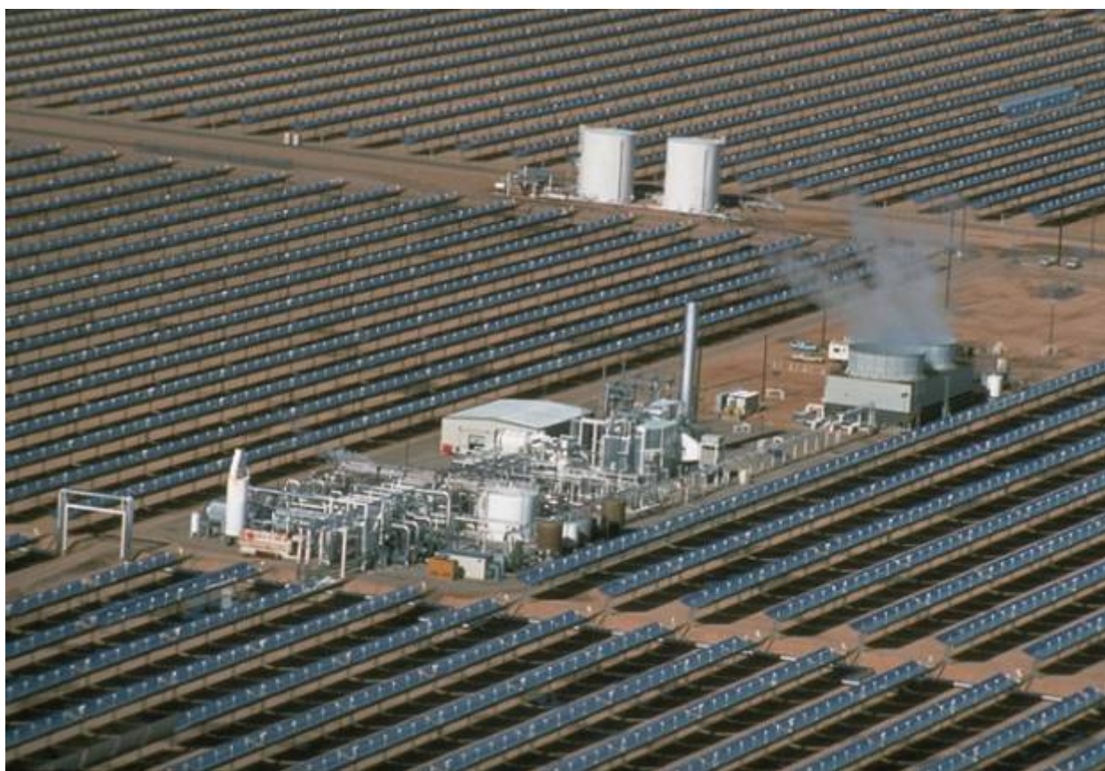
Figure 5-1: Power block of the SEGS parabolic trough power plant in Kramer Junction, US.
