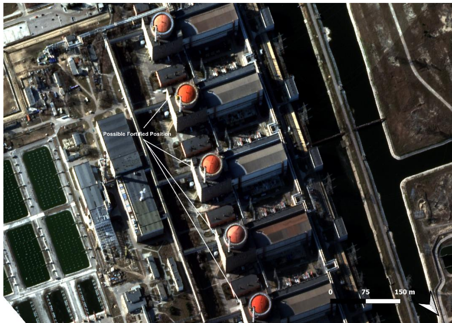
Fig. 24 – Construction of Positions on Reactor Hall Roofs.
