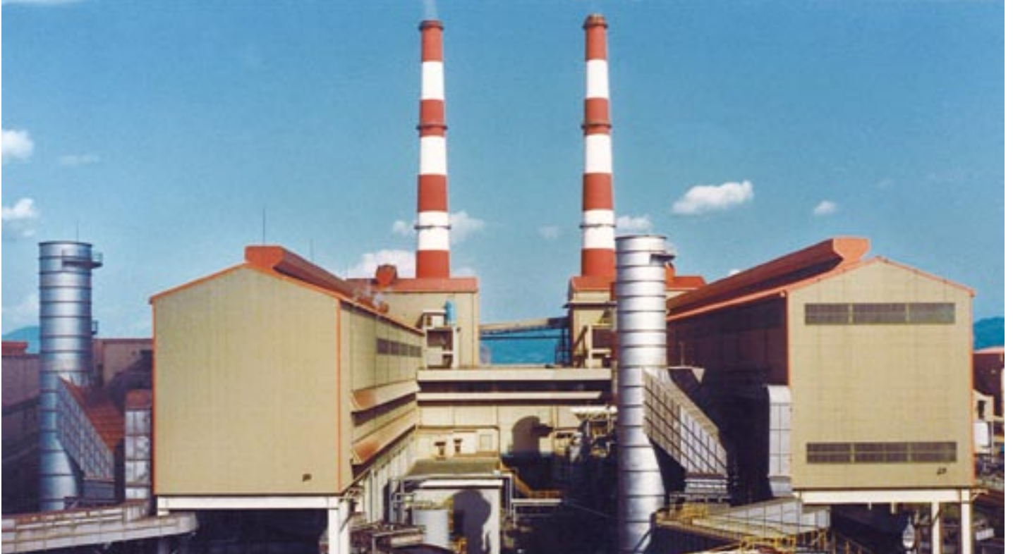
Turnkey sinter plant (4 x 400 m 2 sintering area), Posco, Gwangyang, Korea
