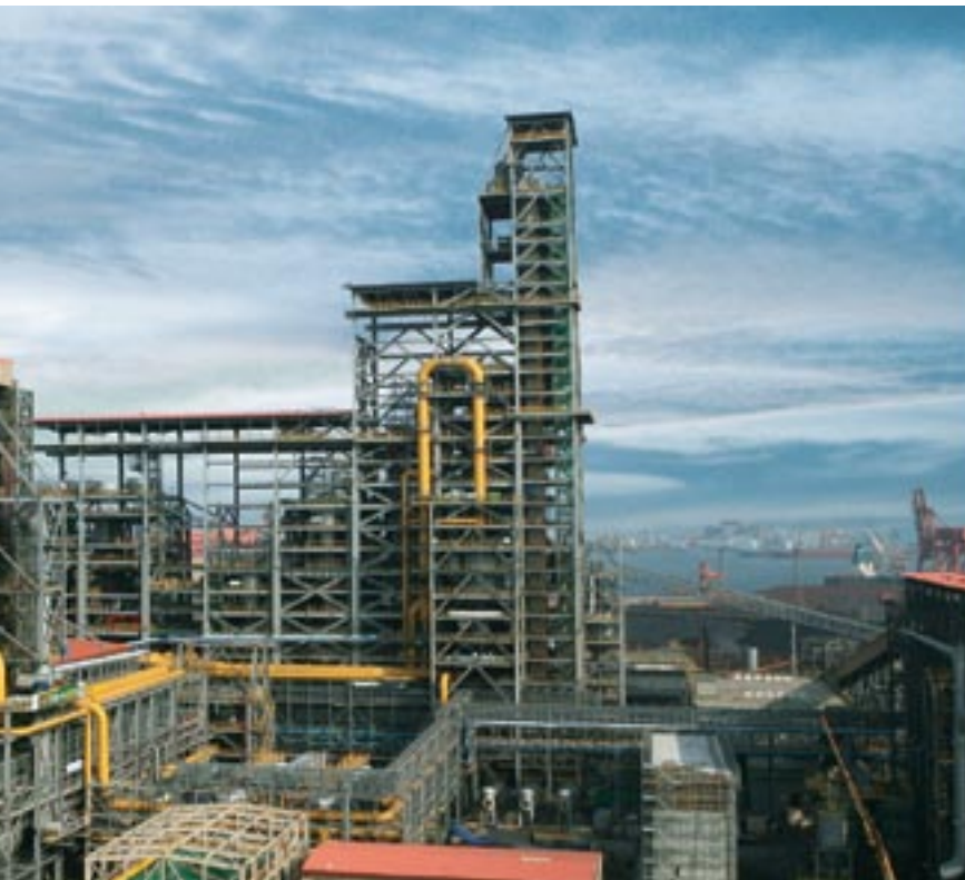
FINEX F-1.5M plant, Posco, Pohang Works, Korea
