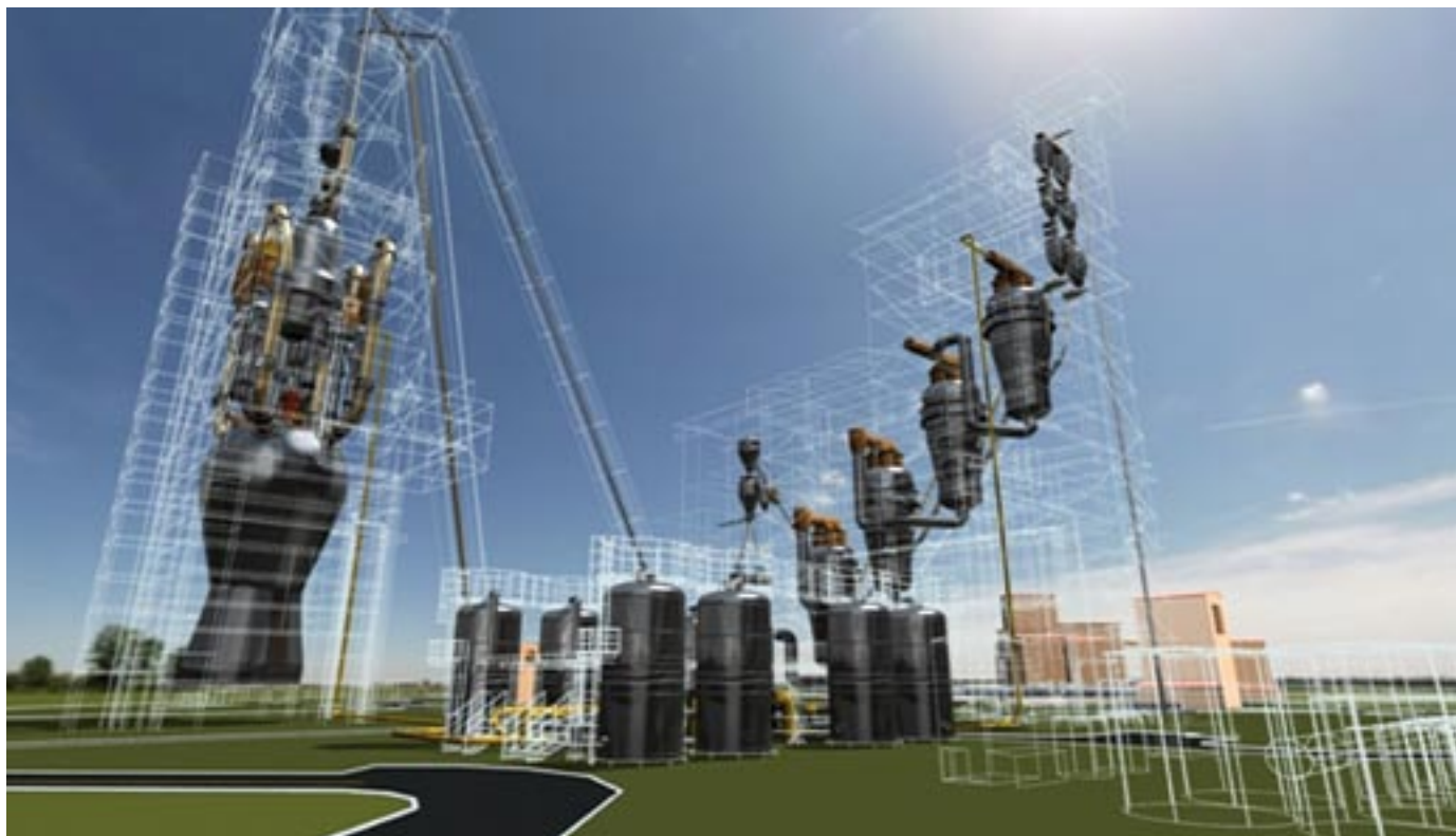
The FINEX smelting-reduction process, a new ironmaking technology based on the direct use of coal and fine ore
