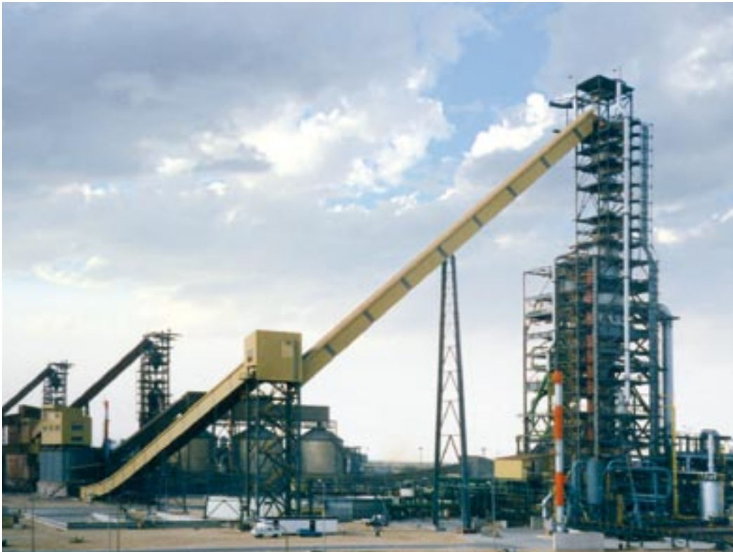
MIDREX plant, Misurata, Libya
